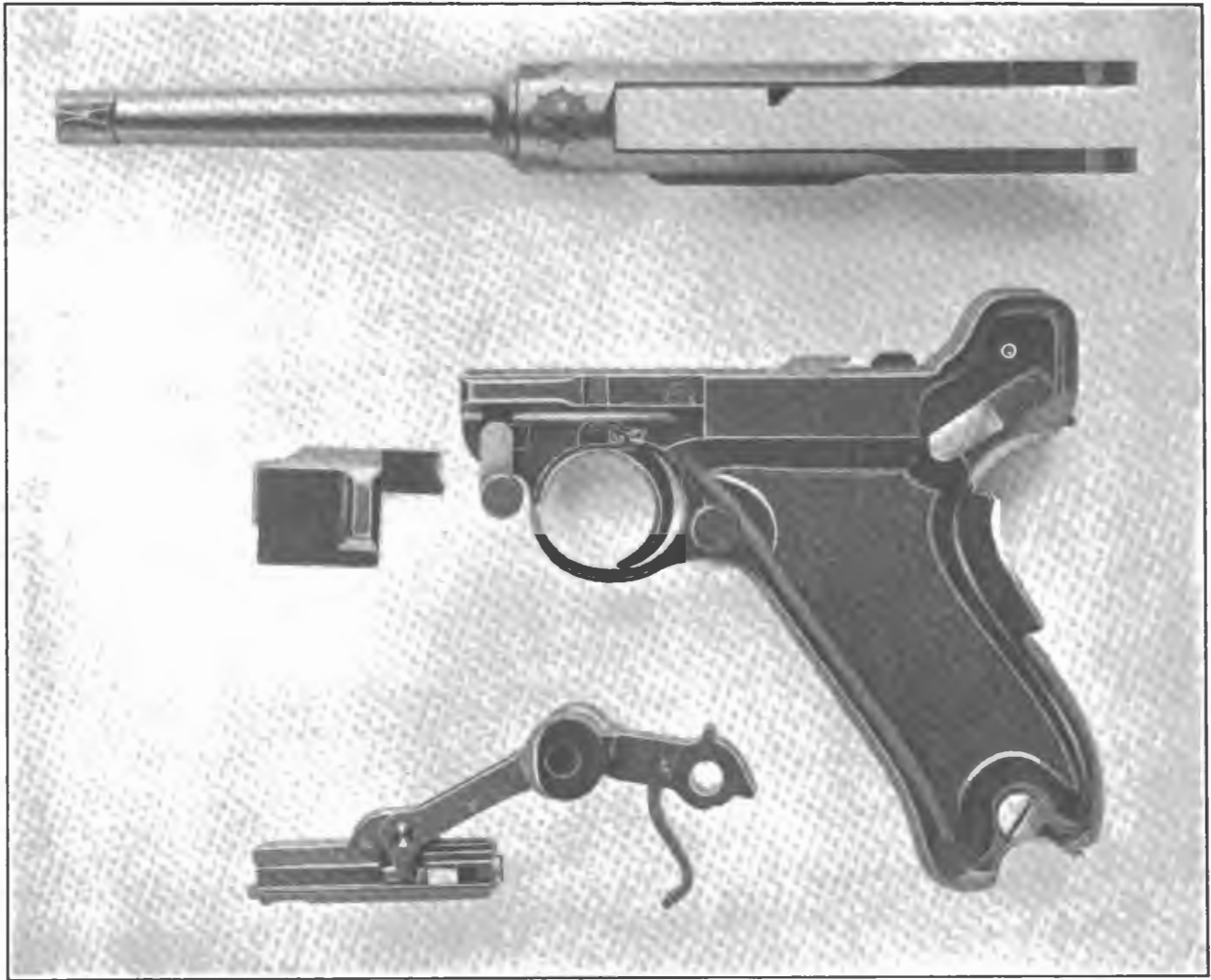
FIG. 3. THE LUGER PISTOL DISASSEMBLED.
